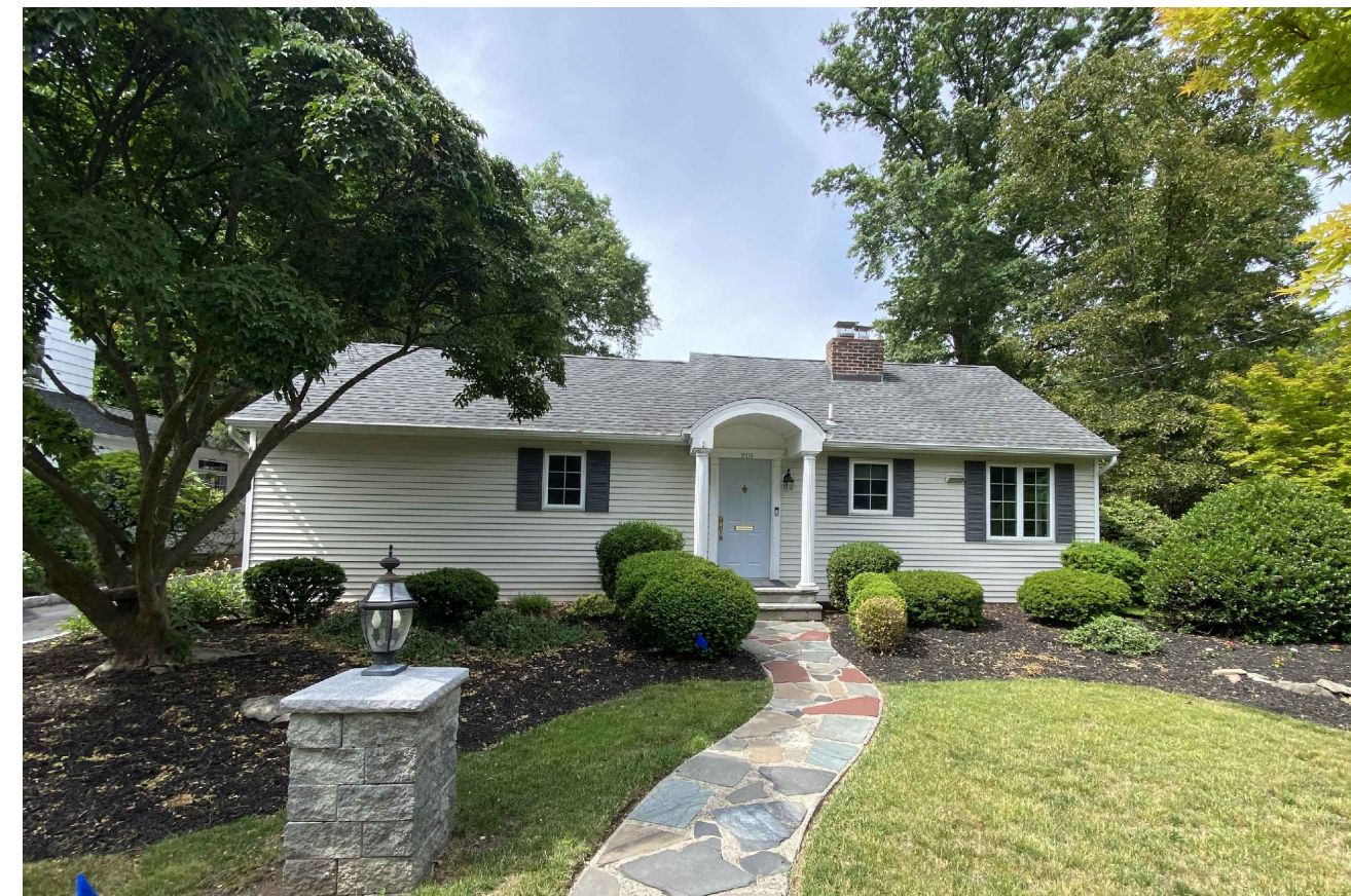
EXISTING CONDITIONS PHOTO
