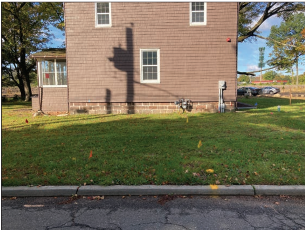
Plate 4.4: View of the John A.L. Zabriskie House showing the north elevation and the location of subsurface utilities (marked).
