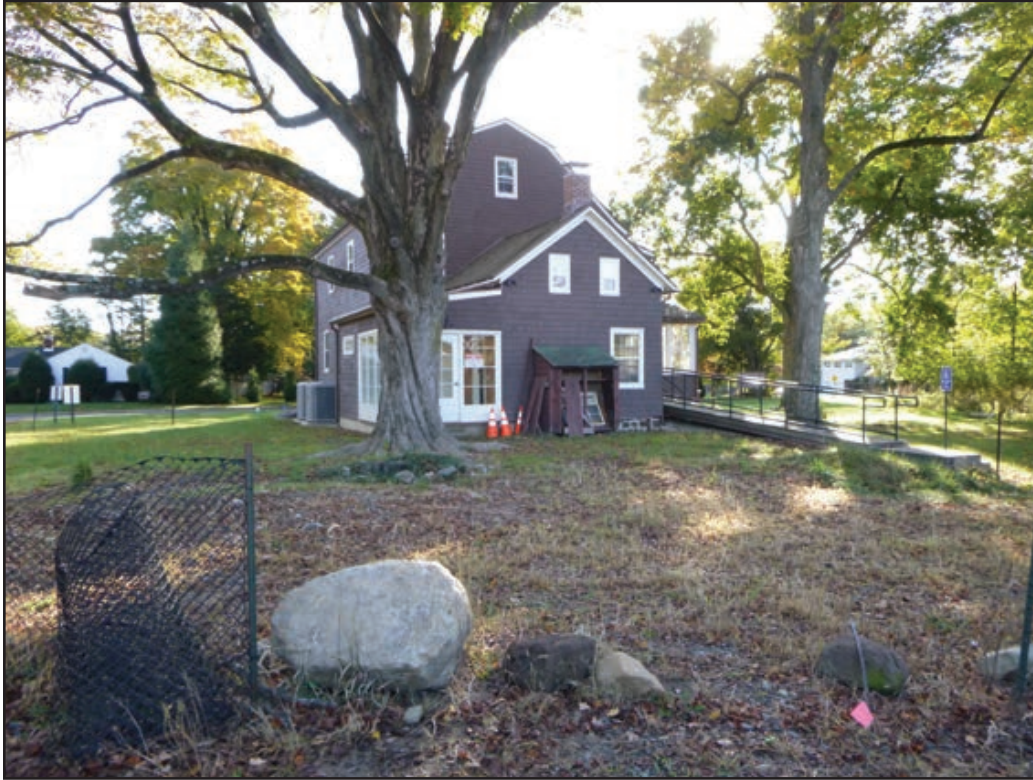
Plate 4.5: View of the John A.L. Zabriskie House showing the north and west elevations, and the fencing and stone boundary of the current yard area.
