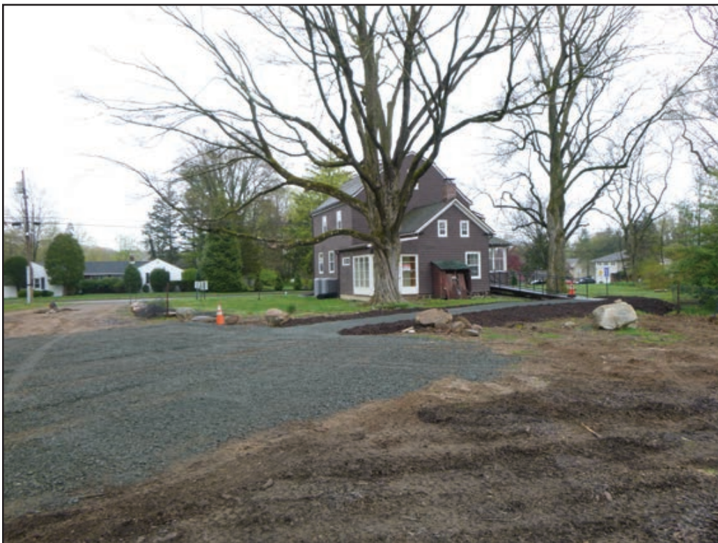
Plate 4.26: Overview of rear of the John A.L. Zabriskie House showing the recent gravel and mulch deposits comprising a portion of the accessible ramp.
