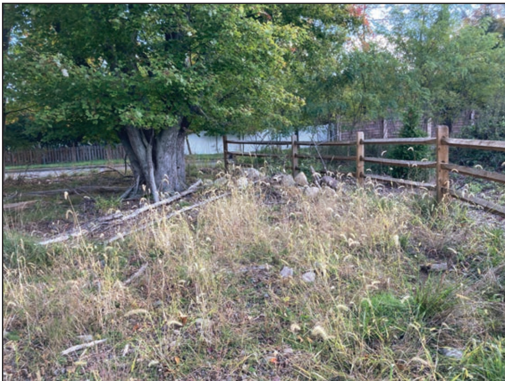
Plate 4.16: View of the southernmost portion of the APE showing installed fencing and piled stone associated with the construction of the berm along Route 17.
