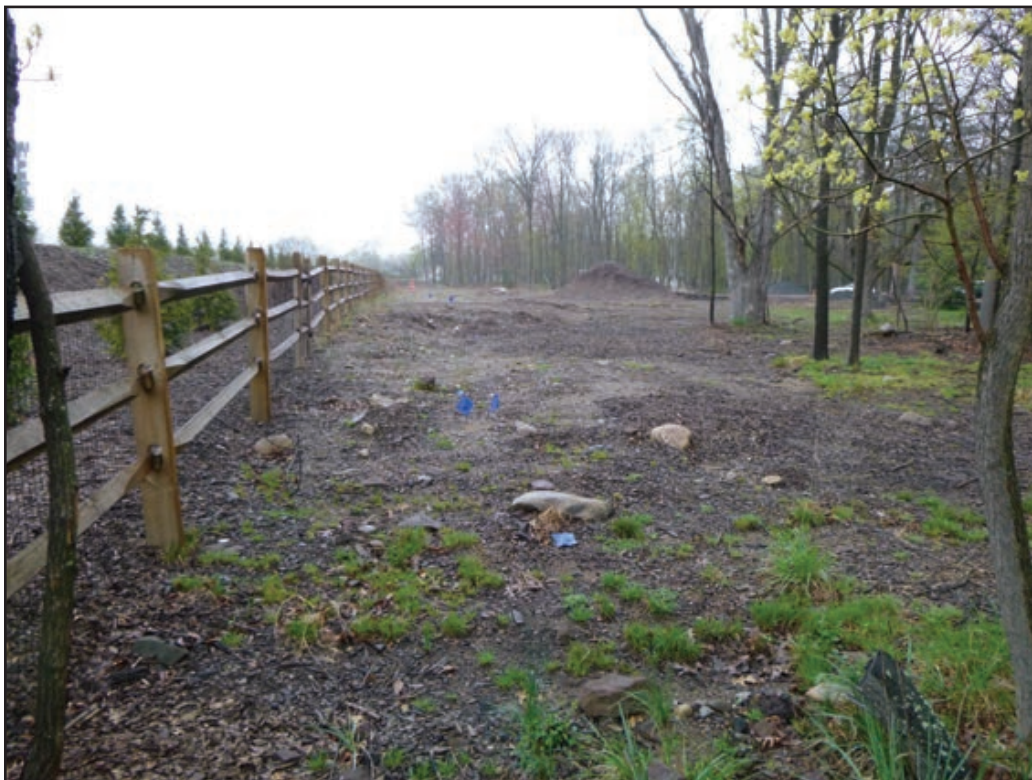
Plate 4.12: View along the NJ Route 17 corridor showing the installed fencing, earth and stone berm, and marked subsurface water utility pipeline.
