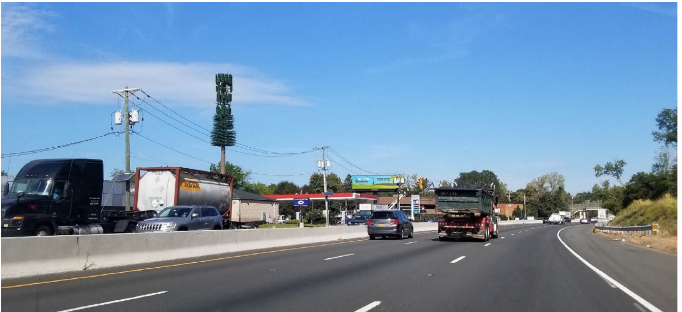
(A-10A: Northbound view from 500 feet)
