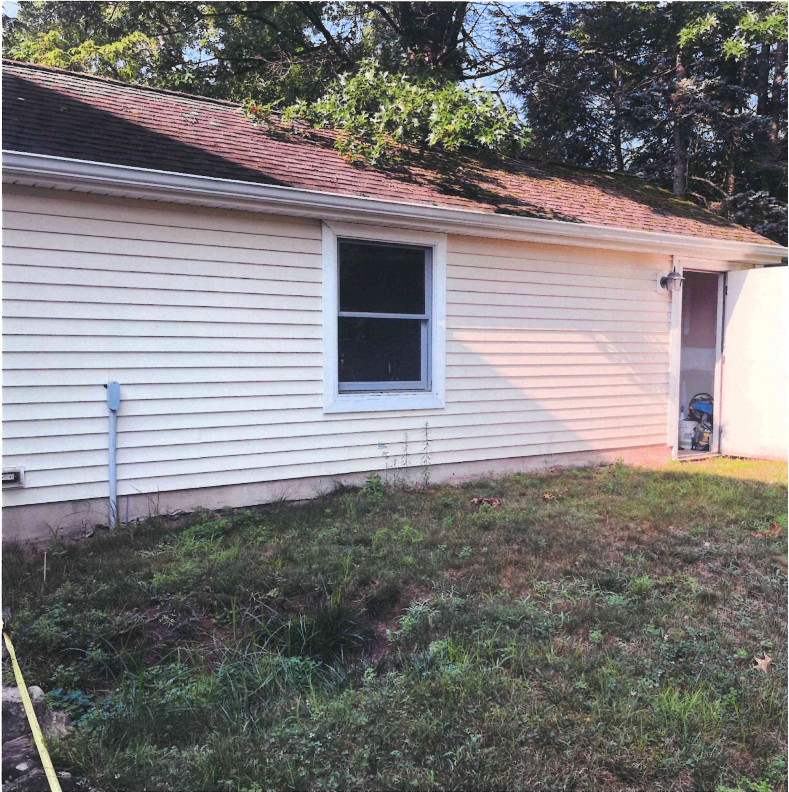
Photo B Lot 10 garage along south side yard.
