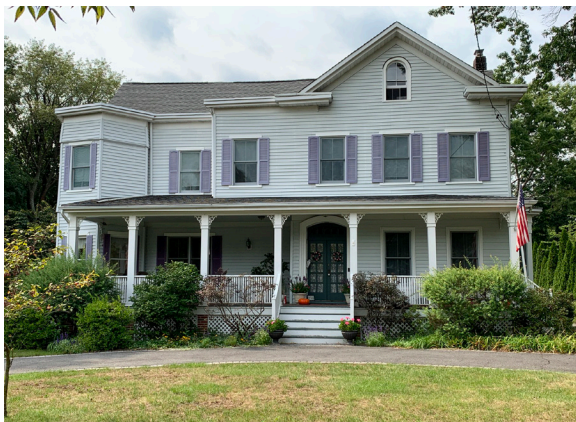
238 South Van Dien Avenue; South Van Dien Avenue Historic District Photo Courtesy of Dianne O'Brien
