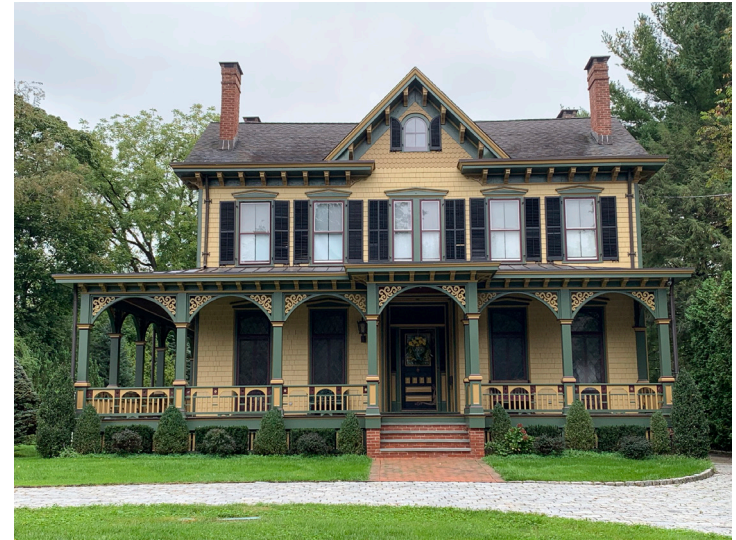
131 West End Avenue; Individually Designated Historic Site Photo Courtesy of Dianne O'Brien
