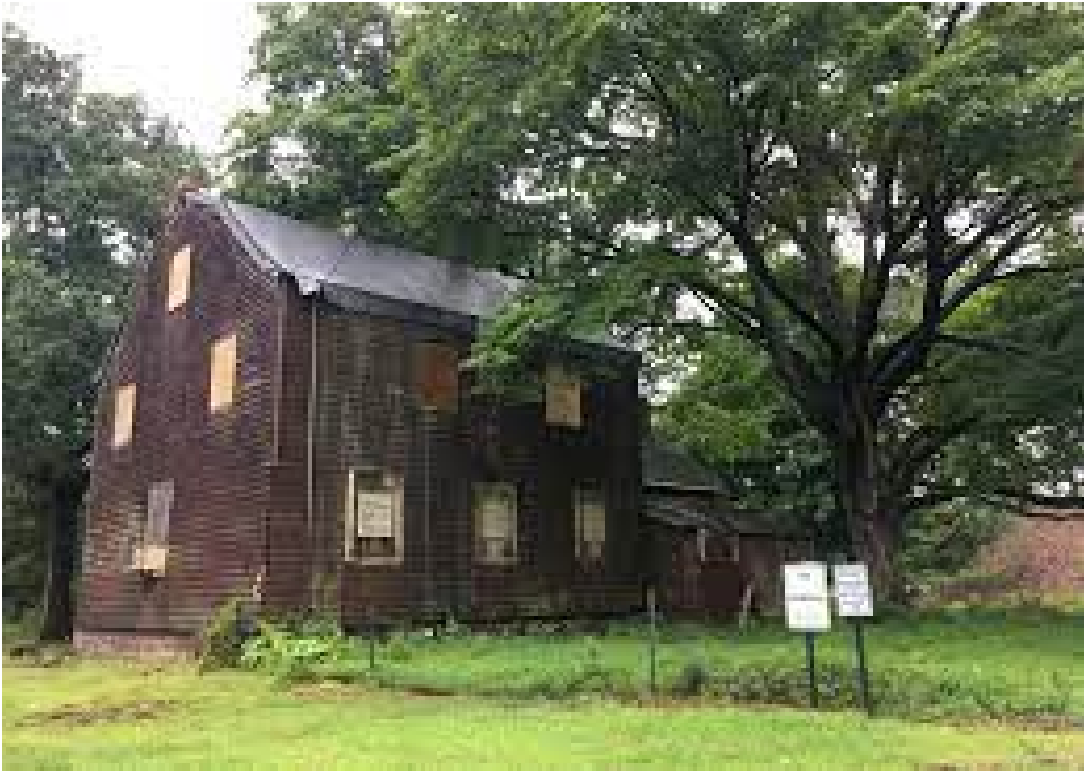
Photo 1 – John A.L. Zabriskie House, Before Restoration
