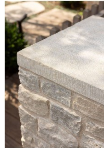
RETAINING WALLS FRONT OF HOUSE
