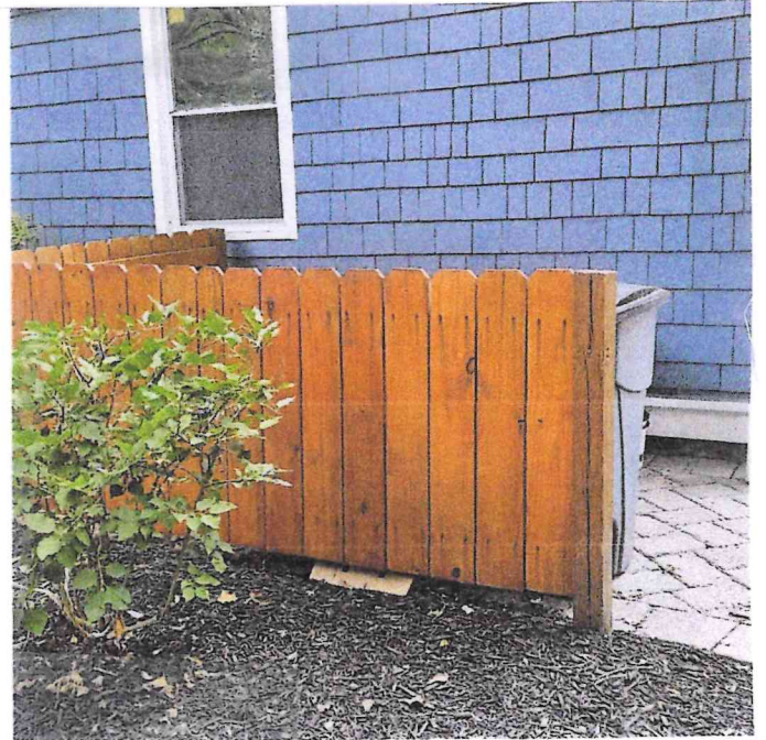
FIG 6 FENCE AROUND TRASH CONTAINERS
