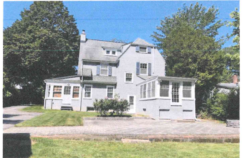
Principal Dwelling - Rear Elevation - 6.25.25
