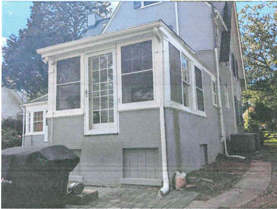
Principal Dwelling - Rear-Side Elevation - 10.15.25
