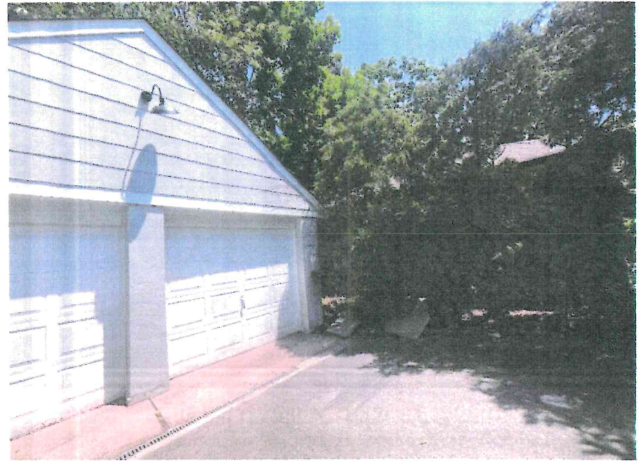
Detached Garage - View towards Right-Side Property Line
